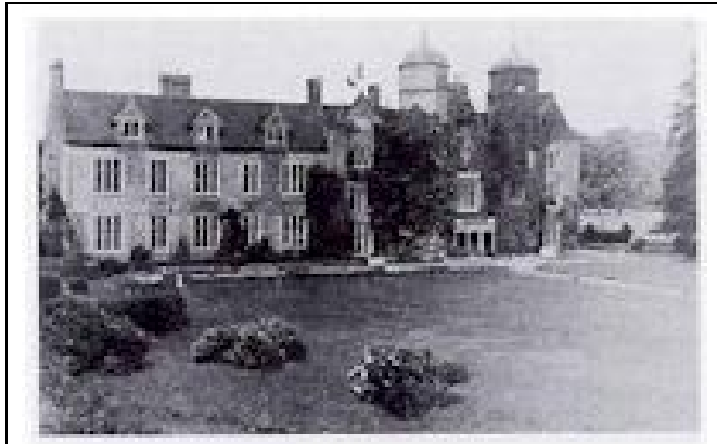
Ribbesford House, near Bewdley
